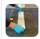
1. Where required, cut butylene tape repair patch to the required size, using supplied Triflex scissors. Loosely place butylene tape repair patch over the affected area, ensuring that the area is completely covered by the repair patch and that it extends past the extent of the defect
