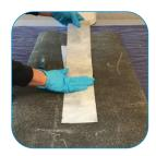
4. Lift the opposite end of the butylene tape repair patch and incrementally peel back the remining protective film to expose the self-adhesive butyl, working along the butylene tape repair patch, pushing it onto the substrate
