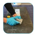
2. With the butylene tape repair patch laid over the area to be repaired, lift one end, peel back and fold the protective film to expose approximately 50mm of the self-adhesive butyl
