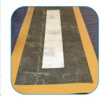
1. Using the supplied 50mm wide Tesa® tape, neatly mask off the area. Where a butylene tape repair patch has been installed as part of the repair, the system should extend approximately 100mm past the extent of the installed butylene tape repair patch. Otherwise, ensure that the Triflex SmartTec Fibre resin extends 100mm past the extent of the defect
