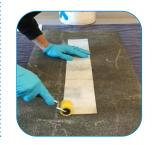
5. When the full area of the Butylene tape repair patch has been adhered to the substrate, work along the patch with the supplied silicone roller to further push and fully bond the butylene tape repair patch onto the substrate
