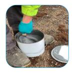
2. Open the drum of Triflex SmartTec Fibre resin using the supplied drum opener and thoroughly stir using the stirring sticks until the resin achieves a uniform consistency. Stirring air and bubbles into the resin should be avoided
