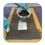
3. Using one of the 75mm paint brushes provided, apply the resin liberally to the area. Consumption should be at 3.00Kg/m<sup>2</sup>
