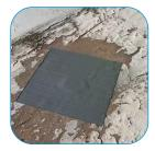
5. Upon completion, immediately remove the Tesa® tape to complete the repair. Place used brushes, gloves and tape in the plastic bags provided for disposal
