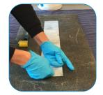
3. Bond the exposed butyl of the repair patch to the substrate and push the tape down onto the surface
