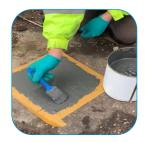
4. The required amount of resin should be adjusted to suit the area required yet retain a consumption of 3.00Kg/m<sup>2</sup>. Brush apply the resin in two directions at 90° to ensure that there are no voids or trapped air present. Neatly complete the resin installation by further brushing across the width of the repair in a single direction towards the installer to create a neat finish
