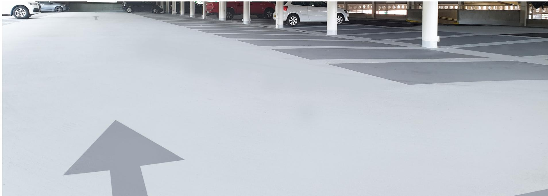
To deal with continued structural movement, Triflex's ETA certified, dynamic crack bridging overbanding was applied on all decks directly above precast reinforced concrete plank joints and above support beam lines.
